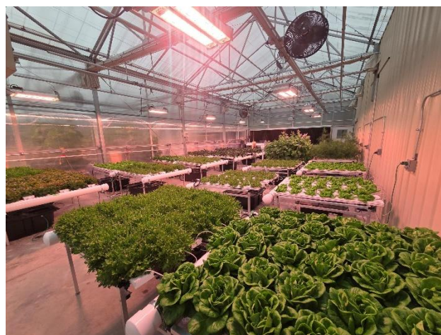
Figure 3. Active greenhouse with LED lights, fans, and cooling pads.
