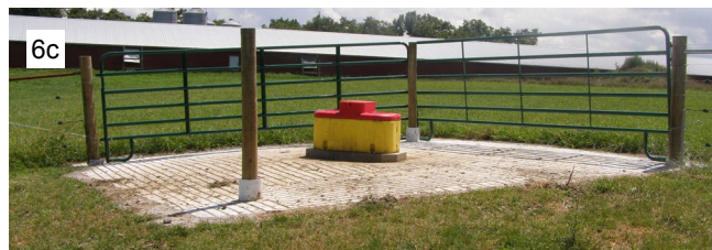
Figure 6. A fenceline water block (6a); a close-up of the fenceline water block using temporary fencing to block access to adjacent pasture (6b); and a water block using movable gates and PVC pipe sleeves set in concrete, allowing posts and gates to be installed or removed to control access (6c). (Photo credits: Matt Booher [6a], Mike Phillips, Rockingham County, Virginia [6b], Cory Williams, Natural Resources Conservation Service [6c].)
