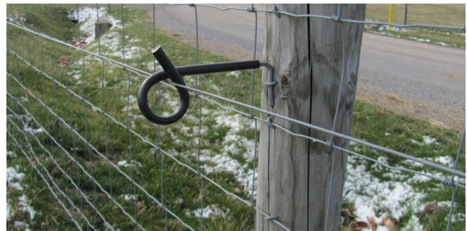
Figure 1. Woven wire perimeter fence with an offset electric wire. (Photo credit: Matt Booher.)
