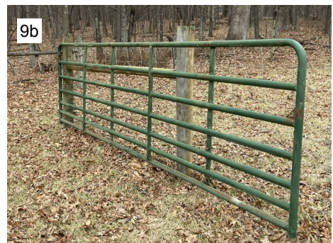
Figure 9. Mounting gate hinges at a slightly offset angle on the anchor post (9a) allows the gates to be opened fully (9b). (Photo credit: Matt Booher.)
