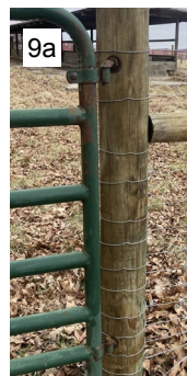
Figure 9. Mounting gate hinges at a slightly offset angle on the anchor post (9a) allows the gates to be opened fully (9b). (Photo credit: Matt Booher.)
