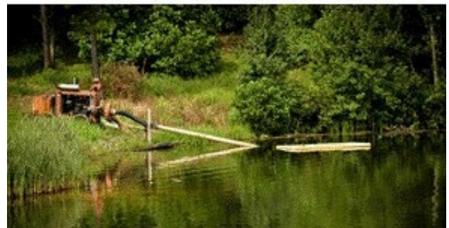
Figure 4. A well head embedded in a concrete pad to provide protection from contamination (top), and a pond and pump used for crop irrigation needs in adjacent fields. (Vallotton; Conservation Fund)
