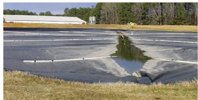
Figure 5. Covered lagoon. (Source: Jay Cheng, North Carolina State University)
