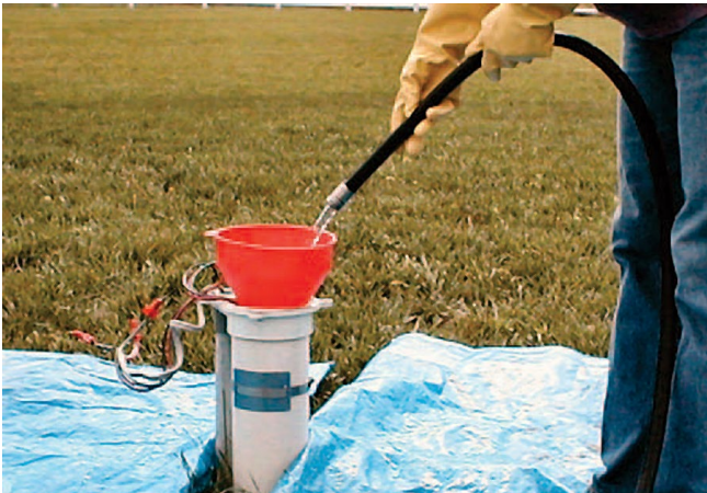
Figura 2. Haga circular el agua en el pozo y lave el interior de la carcasa. Fuente: Departamento de Salud de Minnesota. Source: Minnesota Department of Health. https://www.health.state.mn.us/communities/environment/water/docs/wells/waterquality/disinfection.pdf .
