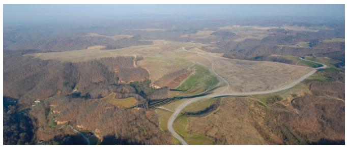
Figure 1. A portion of the Southern Gap Development Area in Buchanan County after reclamation but prior to building development. This site was prepared for industrial use by the mining and reclamation operations; thus, the spoil compaction and road development were cost effective. The paving and utility accesses necessary to enable the site to serve an industrial use were completed as a cooperative effort by the mining contractor and Virginia Coalfield Economic Development Authority (CEDA).
