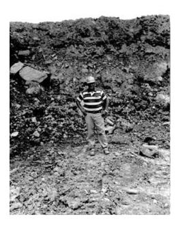
**Figure 5.** The 15-foot surcharge preloading fill at the Red Onion Prison site during surcharge removal. The excavation supervisor is standing on surcharged fill after partial surcharge removal with remaining surcharge material in the background.
