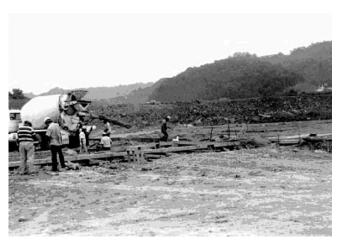
**Figure 6.** Pouring footings at the Red Onion Prison site after site stabilization. The surcharge fill is visible in the background of the photo.
