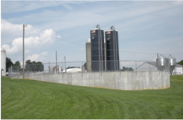
Figure 1. Manure storage structure with a well-kept landscape area.
