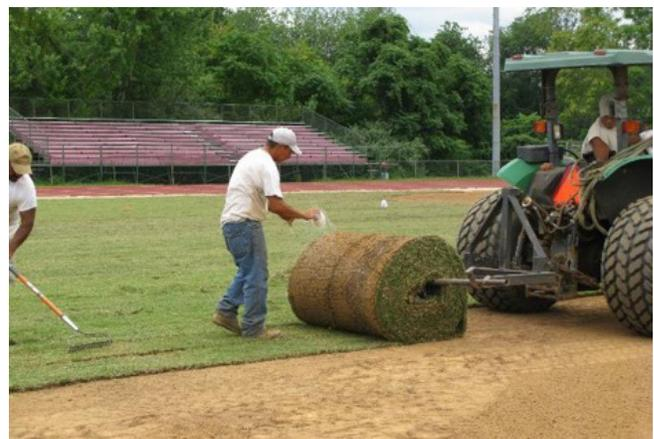
Figure 8. Netting installed for transport and installation of big roll sod is removed at installation. (Photo by author.)
