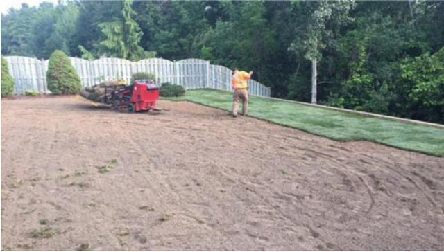
Figure 11. Establish a straight line for sod installation using a sidewalk, driveway, or retaining wall and stagger the seams of the sod as much as possible during installation.
