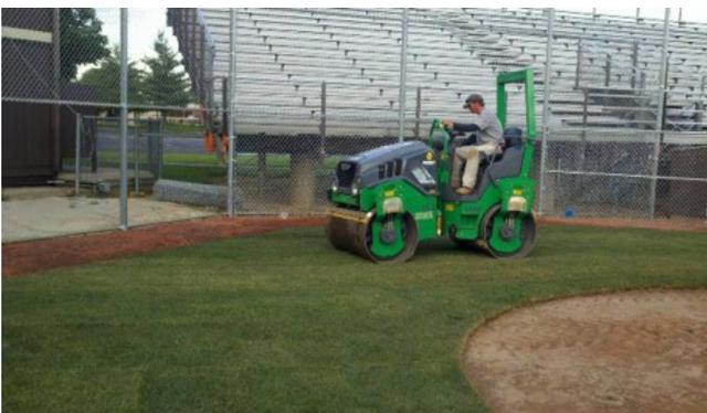
Figure 12. A roller is being used to achieve both sod-to-soil contact and to smooth the playing surface of this baseball field. (Photo by author.)
