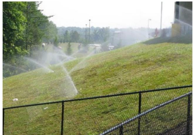
Figure 13. Supplemental irrigation is crucial for successful establishment of a newly installed sod. (Photo by author.)
