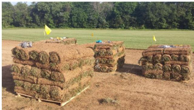
Figure 4. Small roll sod requires no special equipment for handling and installation and can be hauled with the right size vehicle as either individual pieces or as a pallet containing up to 700 square feet of sod. (Photo by author.)
